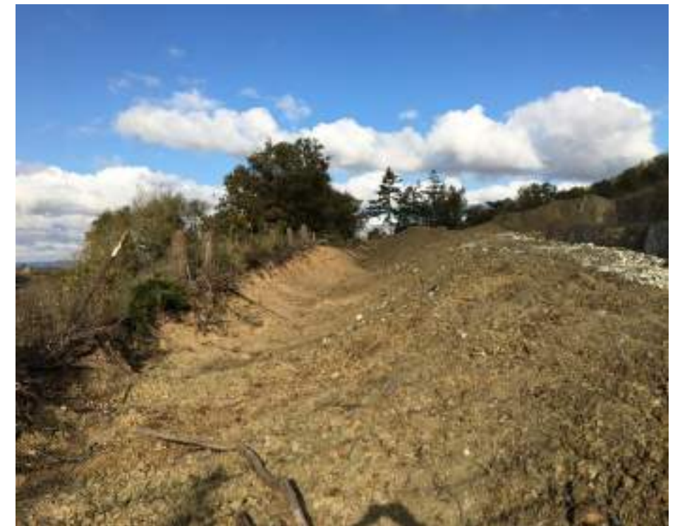
Photograph 8: View looking northern along crest of western excavation. Vegetation has been cleared with good exposure. No indications of tension cracking, deformation or signs of instability.
