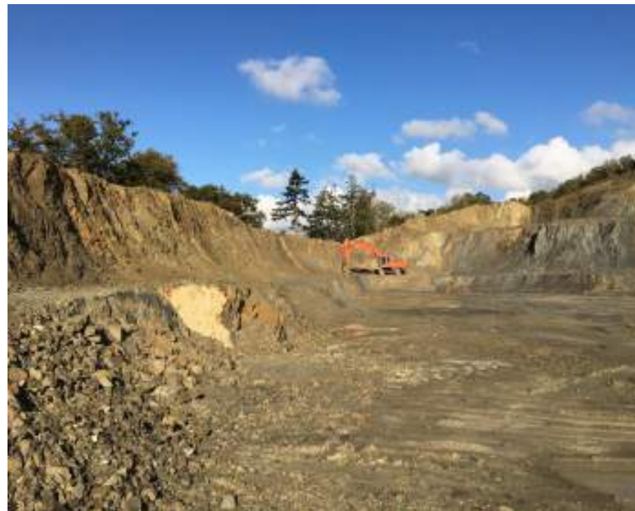
Photograph 7: General view looking north along the western excavation. Some spalling at base of slope but excavation appears stable at 70-80°.
