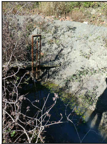
2. Site drain with penstock flow control
