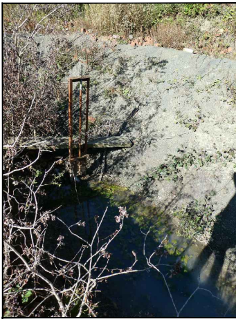
2. Site drain with penstock flow control
