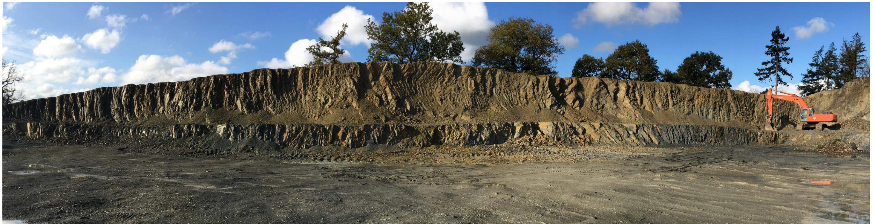
Photograph 5: Panoramic view of western excavation face showing 1.5m high lower face and 2-4m high upper face. Some minor spalling present but no signs of significant instability. Angle of face is variable up to approximately 70-80°. Face is dry with no indications of groundwater seepage.
