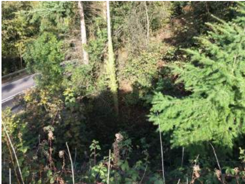
Photograph 12: View looking down into former highways cutting with 50-60° vegetated slopes. No indications of tension cracking or instability although some historical spalling evident at base of slope.
