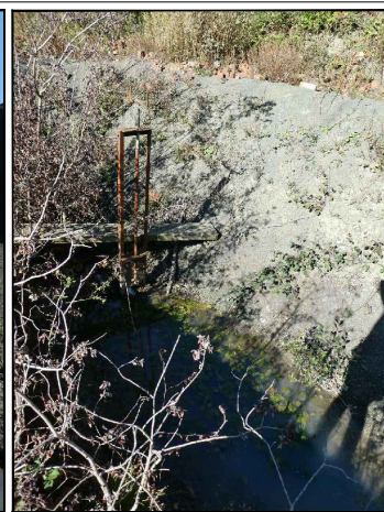
2. Site drain with penstock flow control
